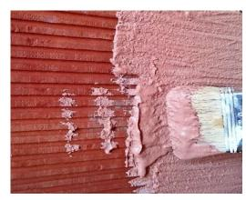
in concrete, lime-based screeds and/or cocciopesto both vertically (walls against the ground or old foundations) and horizontally (tops of facings or exposed parts without roofing); on plasters that are intended to be protected from absorption or water infiltration. Resistant to saline aggression. If necessary, it can be covered with lime finishes or paints.
