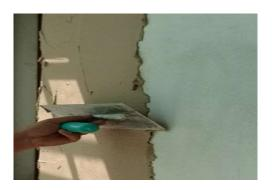
**USE:** The topcoat, very breathable, to be used as a coating or finish, with a fine effect or smoothed according to the process, on cocciopesto plaster, or even as a coloured finishing coating for traditional or premixed plasters; in these cases, test the product on the application surfaces to better verify the final result.
