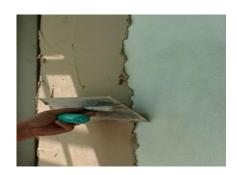
**USE:** The topcoat, very breathable, to be used as a coating or finish, with a rustic effect, on lime plaster or lime-cocciopesto, or even as a coloured finishing coating for traditional or premixed plasters; in these cases, test the product on the application surfaces to better verify the final result. Specific for plaster cycle for renovation of crevice damp.
