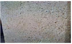
**COMPOSITION:** Hydrated lime (Calce idrata fiore), marble aggregate, siliceous aggregate, natural hydraulic lime, soft-mixed brick cocciopesto.
